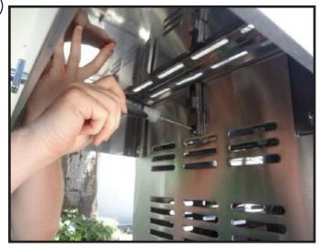
Remove the screw on the center post and loosen the screws on the left and right posts.
