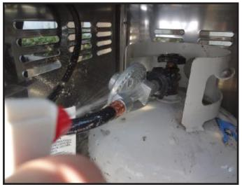
Also apply the soapy water solution to the gas valves you just replaced.
