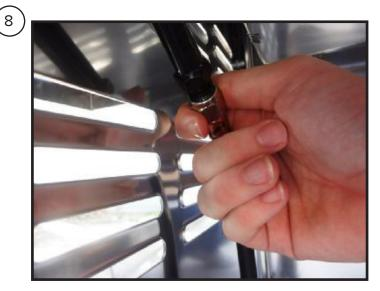
Attach the new regulator gas hose by turning the brass fitting clockwise onto the manifold until it is hand-tight.
