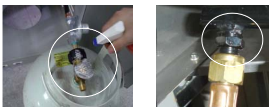
Gas Connection Leak Check
