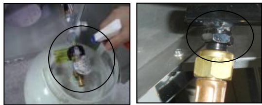
Gas Connection Leak Check
