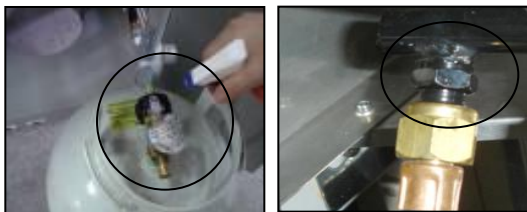
Gas Connection Leak Check
